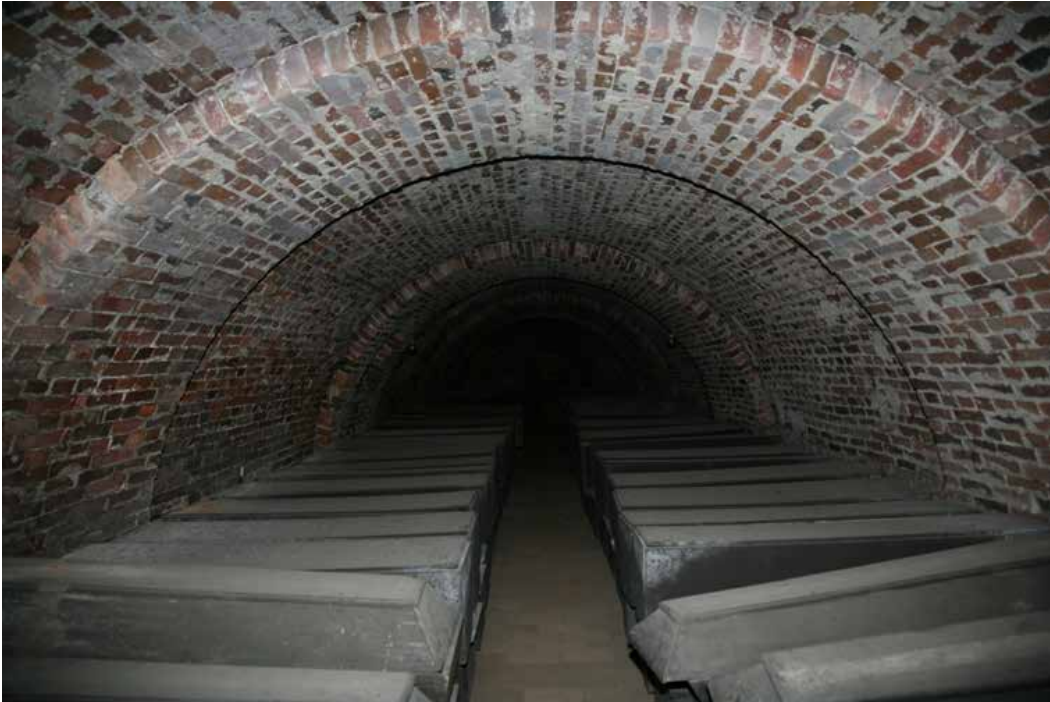
Figure 1: View of interior of the monastery crypt in the former Cistercian church in Lubiąż. Photograph by Martin Mádl
