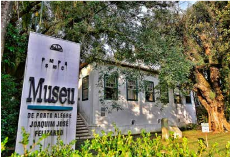
Figure 1: Exterior view of the building of the Museum Joaquim José Felizardo.
