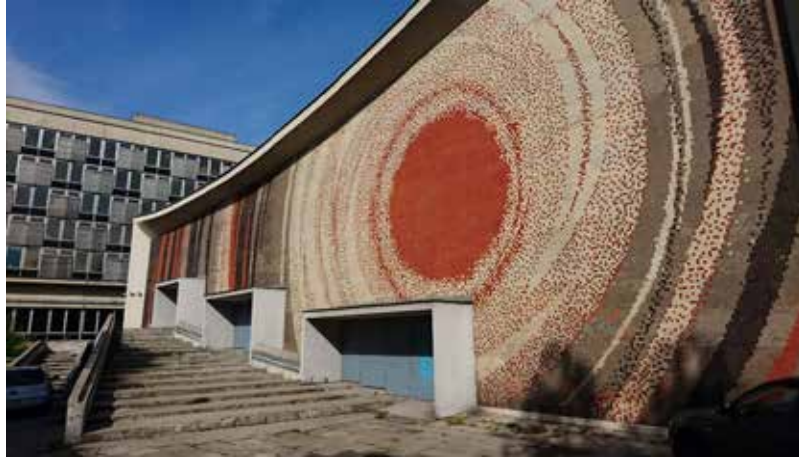
Fig. 2: Rear façade of Kijów by Witold Cęckiewicz after restoration. 2016. Fot. Author
