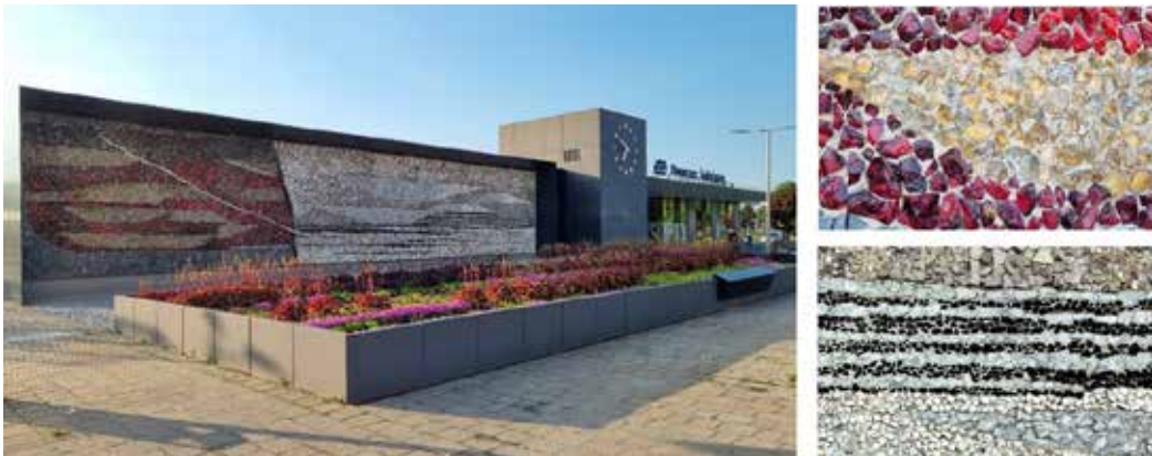
Fig. 7: Oświęcim – new building of the railway station with mosaic by Kazimierz Gąsiorowski. 2021. General view and detail of restored artwork. Fot. Author
