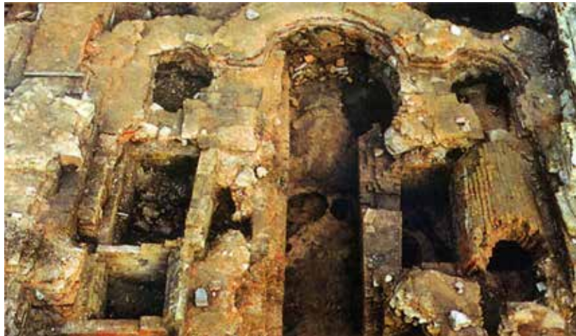
Fig. 1: Fragment of ancient foundations of St Michael's Golden-Domed Cathedral. Photo: [in:] Collection of the Ukrrestavratsiia Corporation
