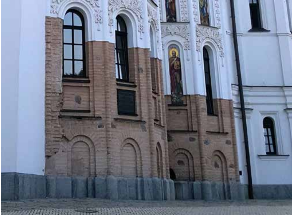
Fig. 6: Reconstruction of old masonry techniques on the apses of the Dormition Cathedral. Photo by D. Kuśnierz-Krupa, 2019
