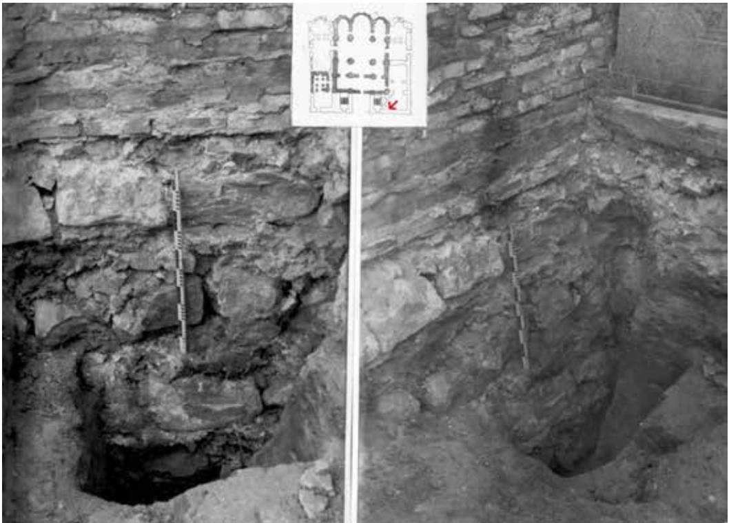
Fig. 4: The Dormition Cathedral. Excavation site no. 20 b. Pit in the north-western corner of the southern vestibule to determine the footing level. Photo: [in:] Collection of the Ukrrestavrtsiia Corporation.
