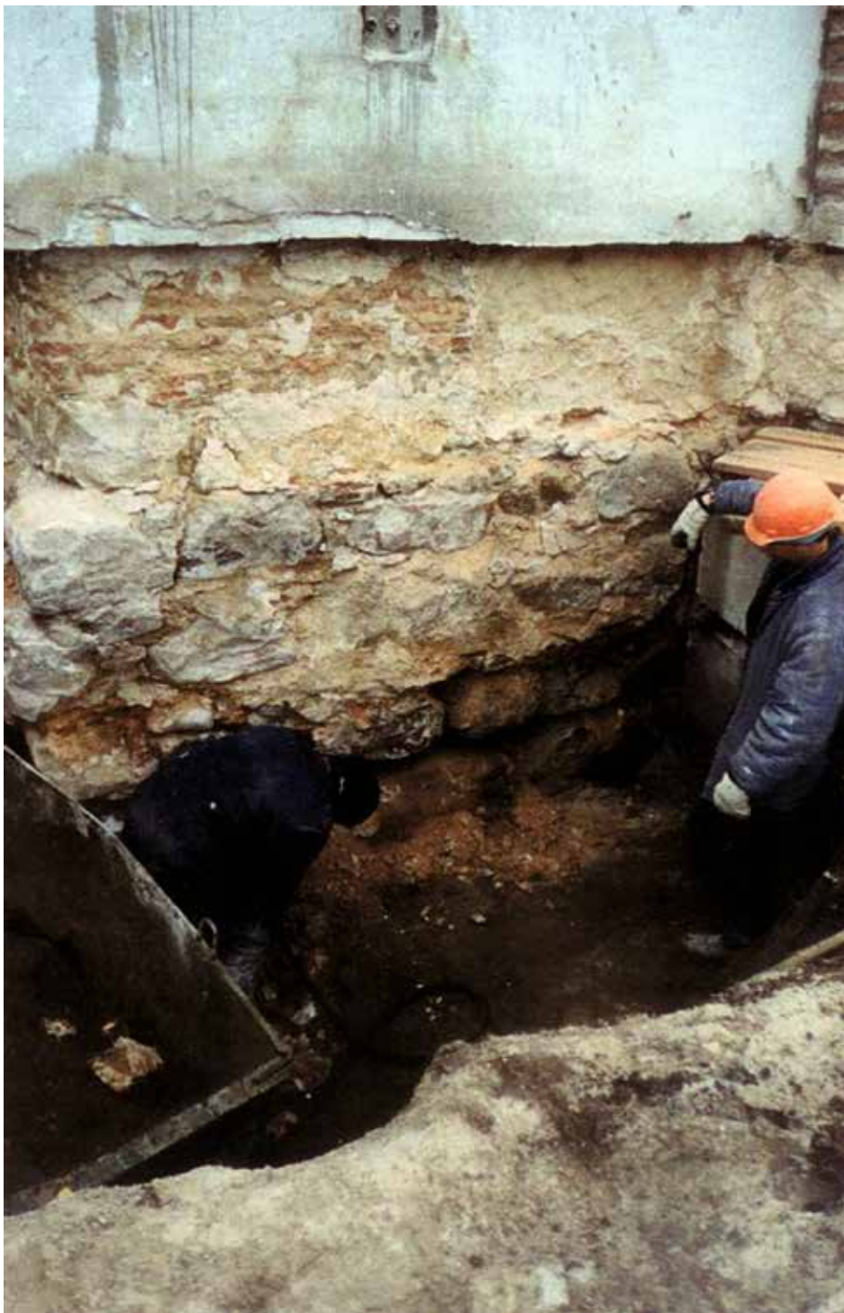
Fig. 5: Fragment of ancient foundations of the Dormition Cathedral. Photo: [in:] Collection of the Ukrrestavratsiia Corporation
