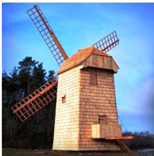
Fig. 26: A windmill from Ruska Wieś in the Museum of Folk Architecture – Ethnographic Park in Olsztynek; state as of January 2022; source: https://muzeumolsztynek.pl/wiatrak-z-ruskiej-wsi-zostal-wyremontowany/ [accessed: August 24, 2022].
