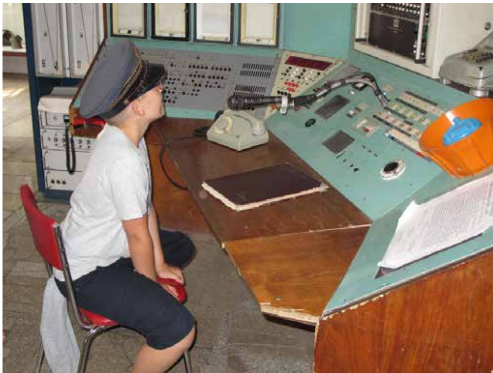
Fig. 8: Control panel – coal mine in Nowa Ruda (Photograph: W. Zglobicki)
