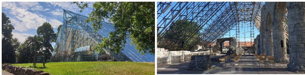
Fig. 7-8: View of the ruins of the Hamar Cathedral covered with a modern glass structure. Photo by Dominika Kuśnierz-Krupa, 2024.
