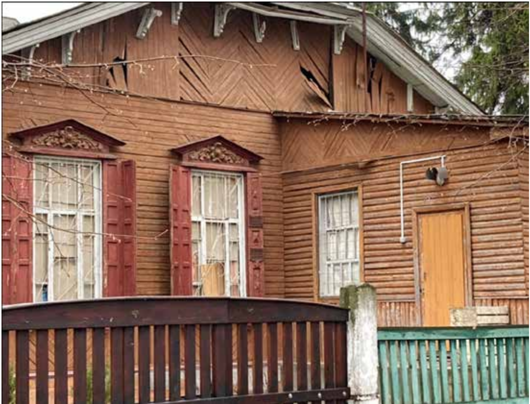
Figure 6: Damage to the end facade of the “wooden Art Nouveau” style mansion. Photo by A. Hlushchenko
