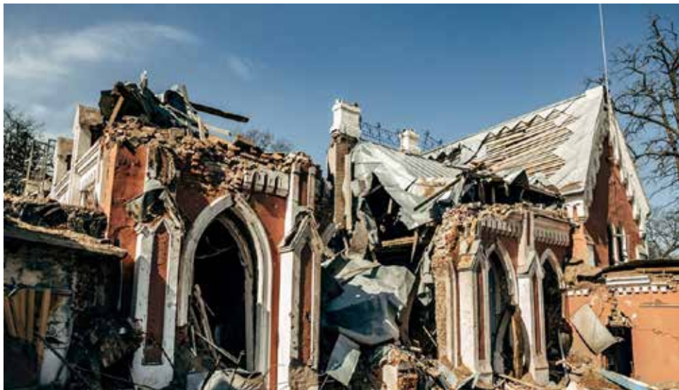
Figure 4: A fragment of the ruined courtyard facade of Tarnowski Mansion. Photo by A. Hlushchenko, 2022
